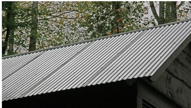
*Figure 21: Corrugated steel roofing*
