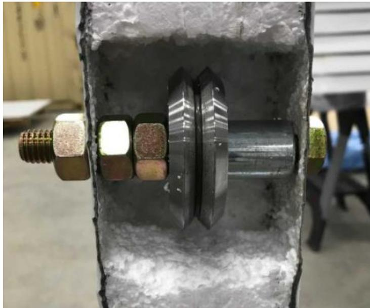
*Figure 53: V-Wheel installation within PermaTherm wall panel*
