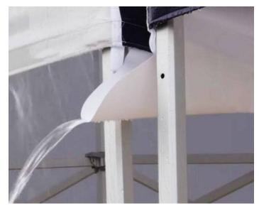
**Figure 36 :** Tent Gutter System In Action (Custom Tents, (n.d.))
