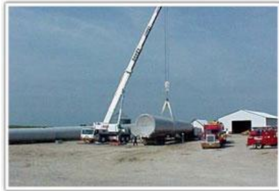
Figure 4.9: Transporting a tower Segment (Lee Wind Energy, 2011)
