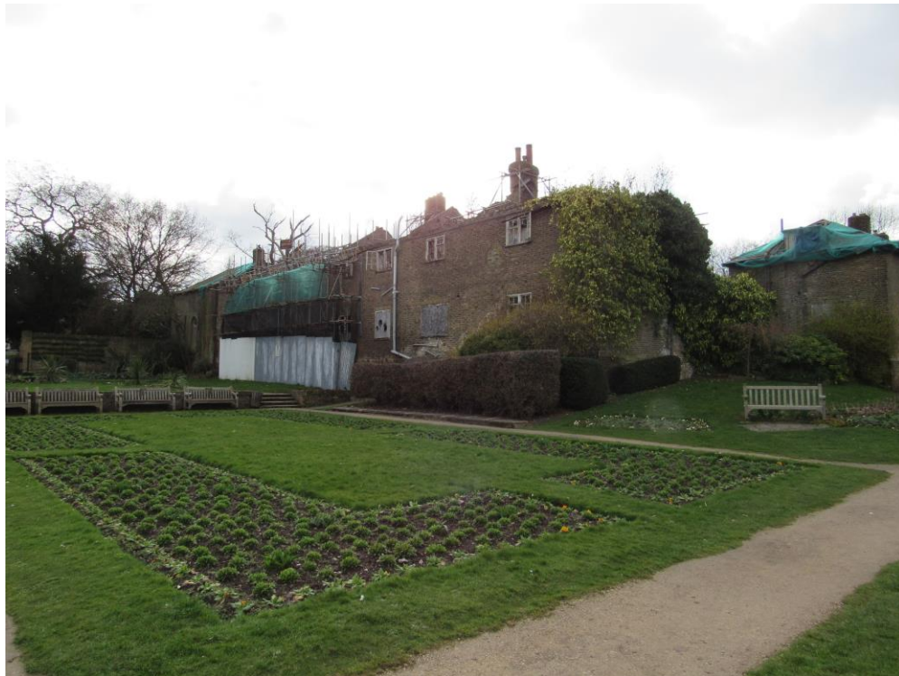
Figure 9: The stables after the 2011 fire.
