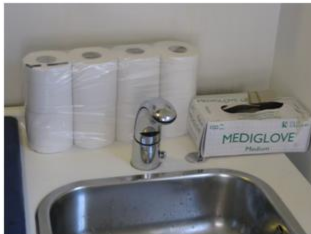
Figure 18: Motion-activated water tap
