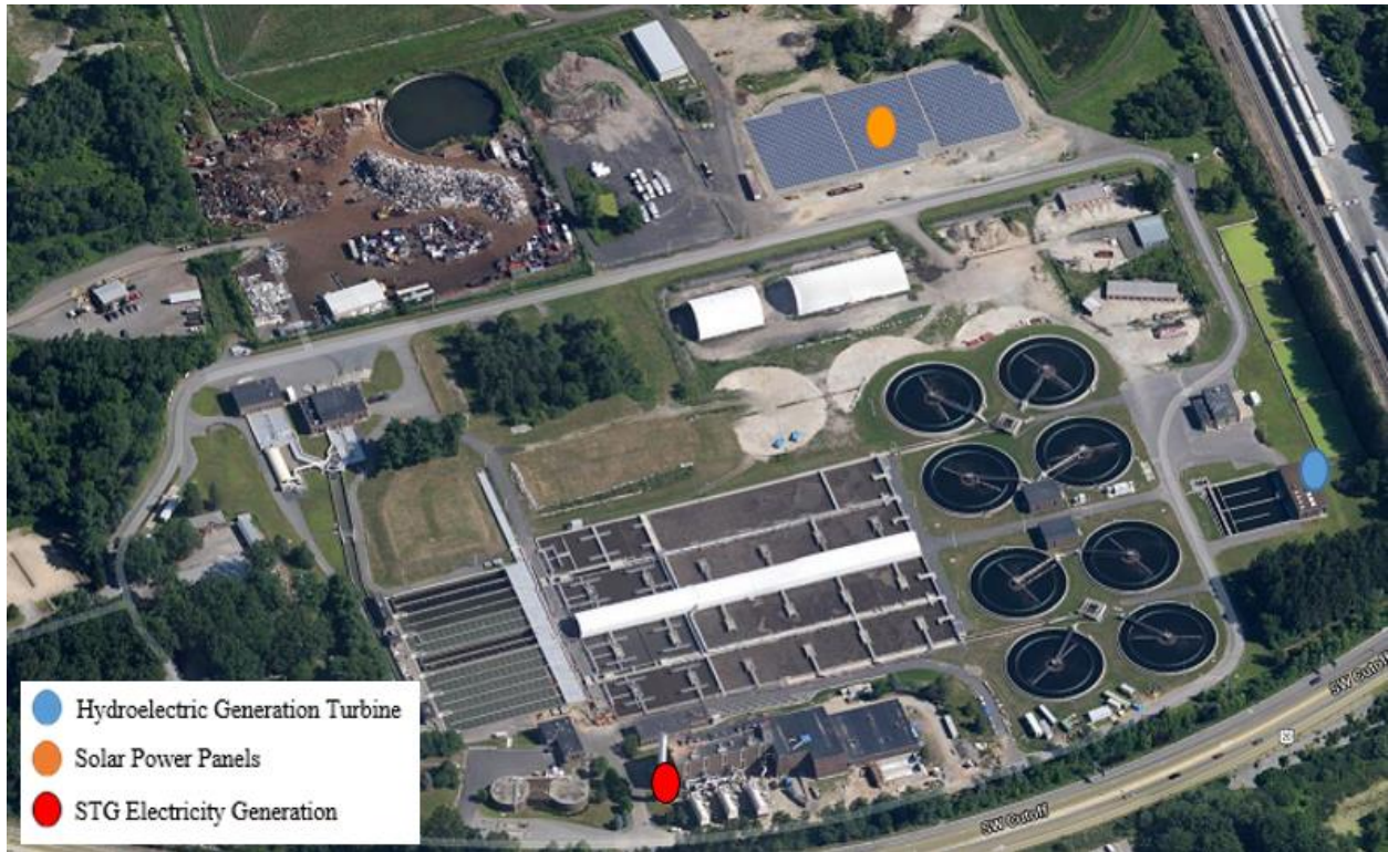
Figure 12 - Potential Energy Reclamation Systems at UBWPAD
