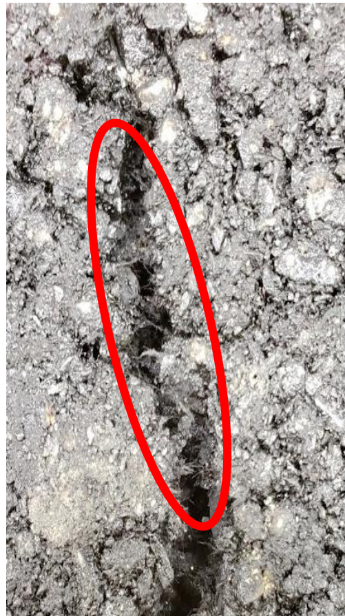
Figure 33: Fiber Bridging in Asphalt Sample
