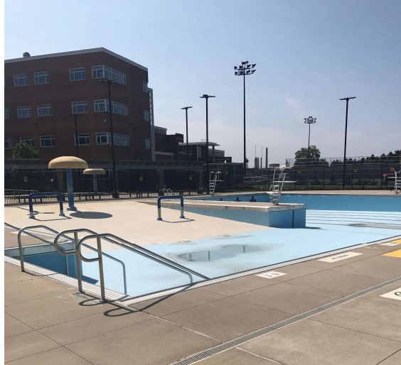
Figure 7: Vietnam Veteran's Pool. Pictured is the Vietnam Veteran's Pool, a public swimming pool run by the Commonwealth of Massachusetts, by the Department of Conservation and Recreation (DCR). Also seen in the background is Chelsea High School.
