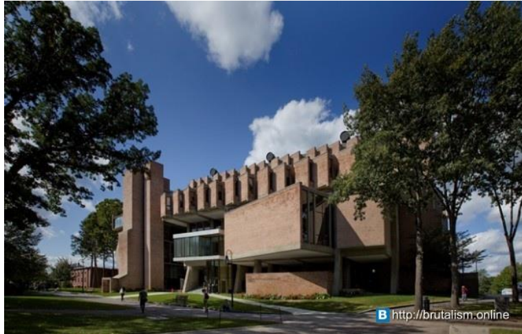
Figure 3: Exterior photograph of Goddard Library.
