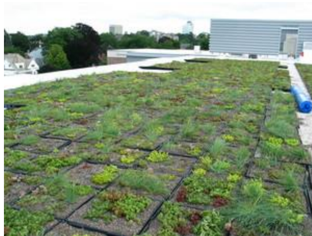
Figure 6: Grid layout of planters on East Hall's green roof.
