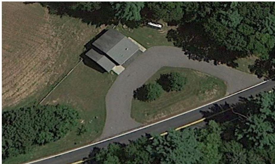
Figure 33. Aerial view of Well 5 and 6 (Google Maps, 2014)
