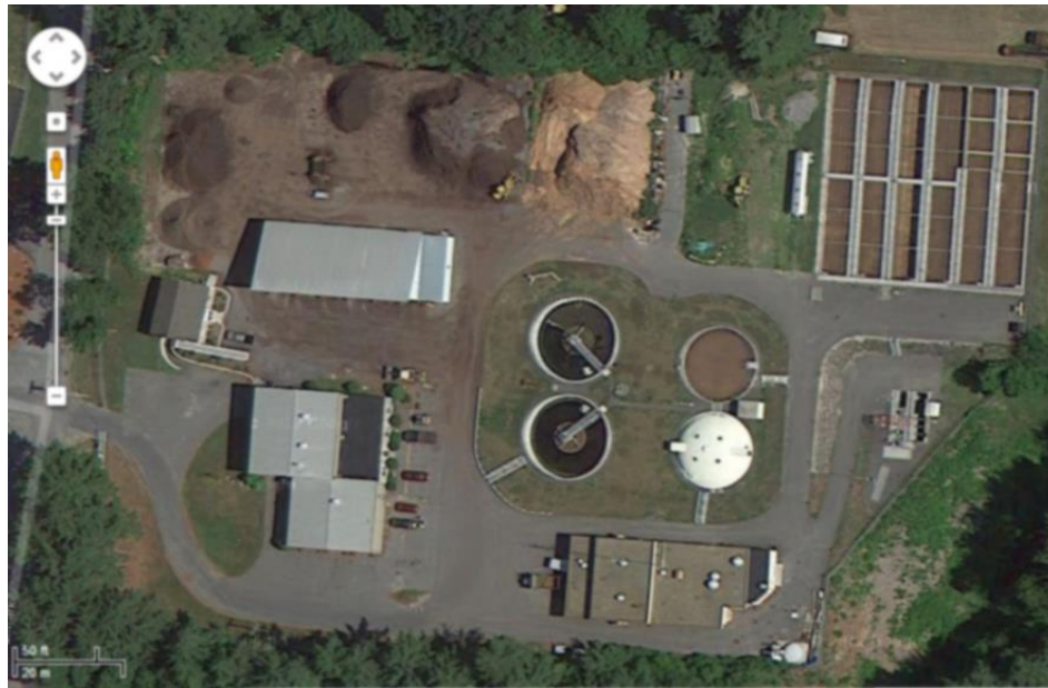
Figure 8. Pepperell Wastewater Treatment Facility Satellite View (Google Maps, 2014)
