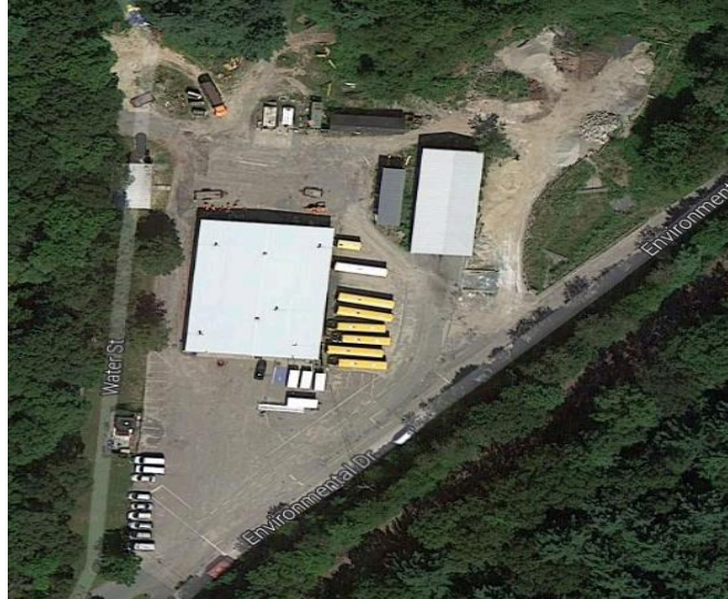
Figure 32. Aerial View of the Millis DPW Administrative Building & Well 1 (Google Maps, 2014)
