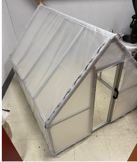
Figure 37: Finished Greenhouse with Polyethylene
