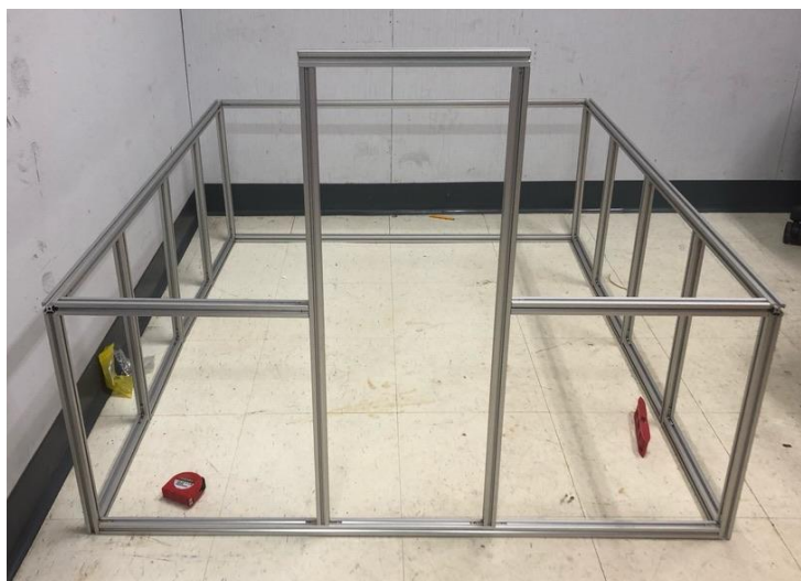
Figure 30: Greenhouse Frame after Day One of Building
