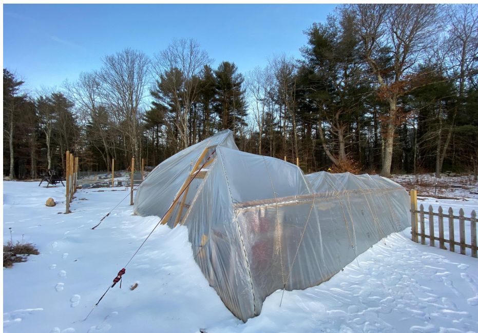
Figure 1: Previous Greenhouse Collapse
