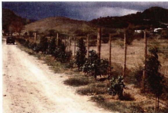
Figure 7: Example of improper fence line spacing of 5 ft.
