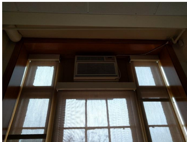
Figure 30: Solar Shade in Kaven Hall
