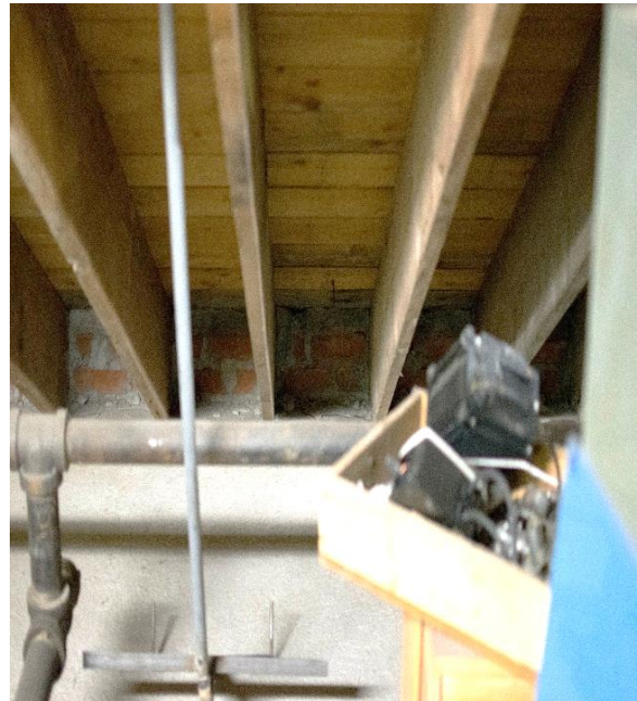
Figure 22: Attic of Kaven Hall Brick Edge
