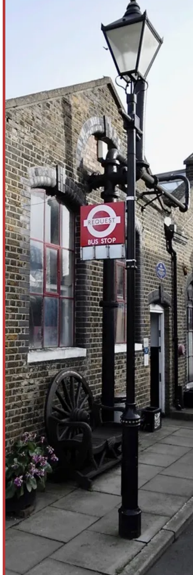
Outside of the Main Pumphouse
