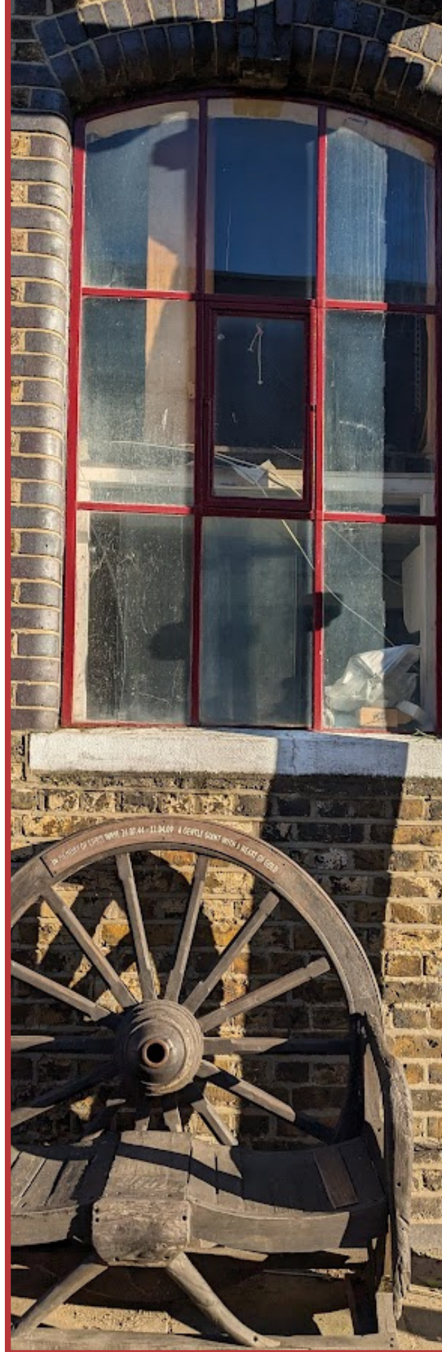
Outside of the Main Pumphouse
