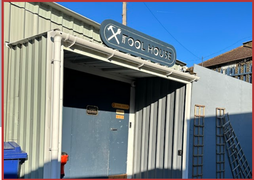
Exterior of the Tool House
