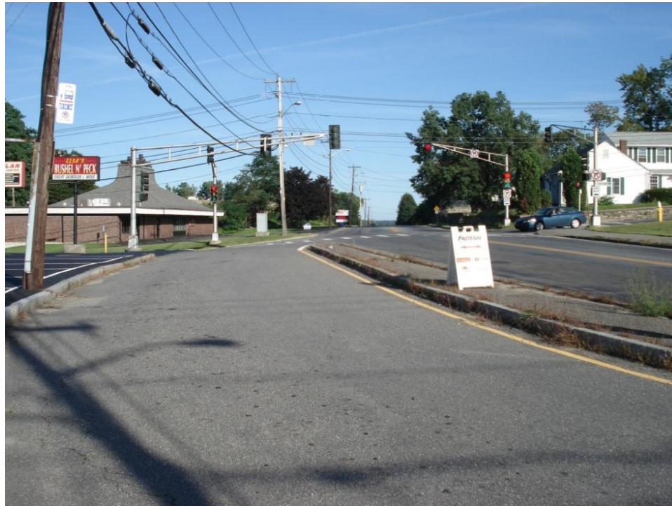
Figure 4: Bus Staging Lane off East Mountain St.
