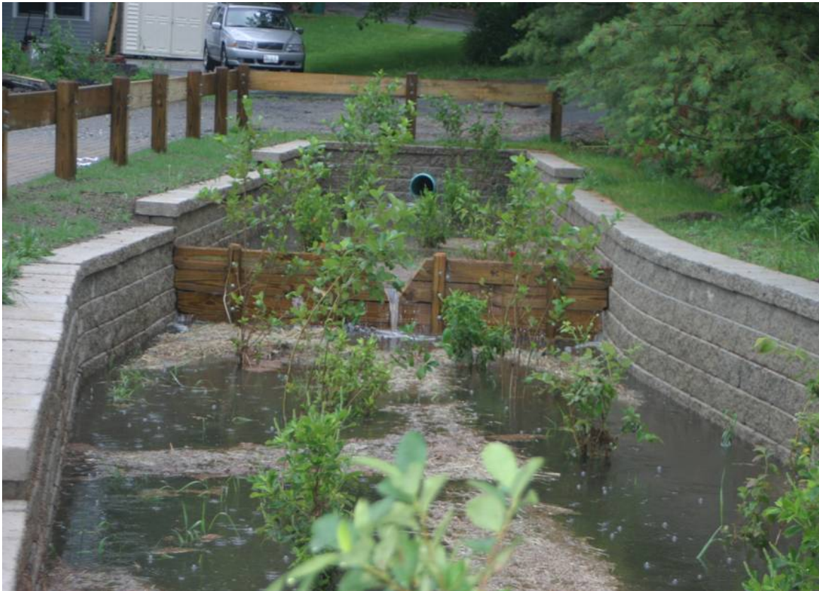
Figure 4.1.2: Cascading Vegetative Swale at Long Lake (Danos, 2006, p.46)
