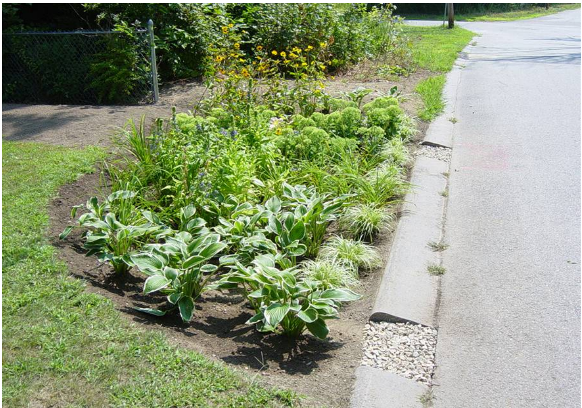
Figure 4.1.3: A Rain Garden near Long Lake (Danos, 2006, p58)
