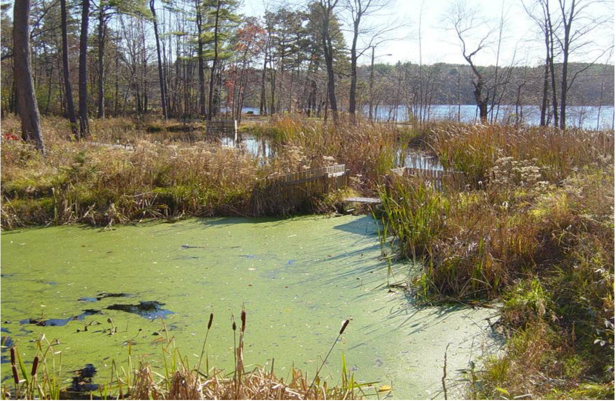
Figure 4.1.1.2: Man-made storm water wetland at Long Lake (Danos, 2006, p26)
