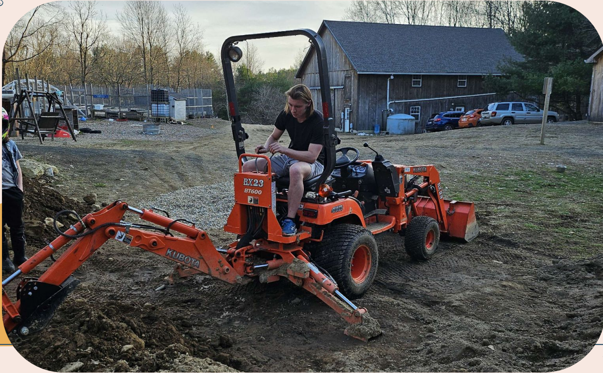
Figure 52: Ethan using the backhoe to clear dirt from the excavation site
