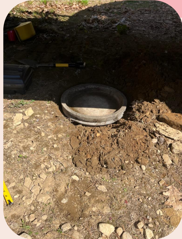
Figure 47: Image of the initial construction of the frog cave.
