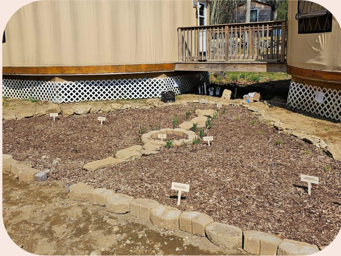
Figure 59: A photo of the completed rain garden with the frog cave in the background.
