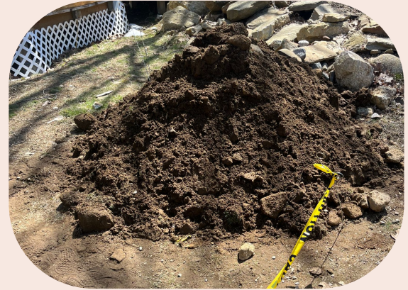
Figure 38: Clay rich soil excavated from the garden site
