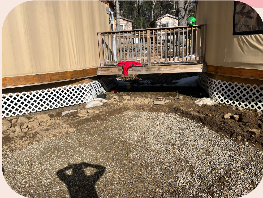
Figure 53: Image of the excavated garden with 1 ½" gravel layer.
