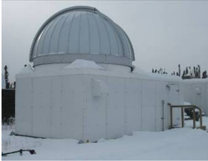
Figure 5: Optics Shelter and Dome
