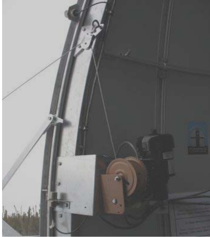
Figure 15: Lower shutter control motor and limit switch
