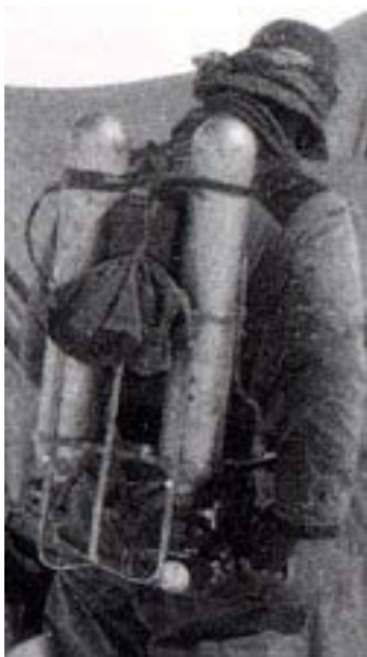
Figure 30 - Intial Oxygen Systems
