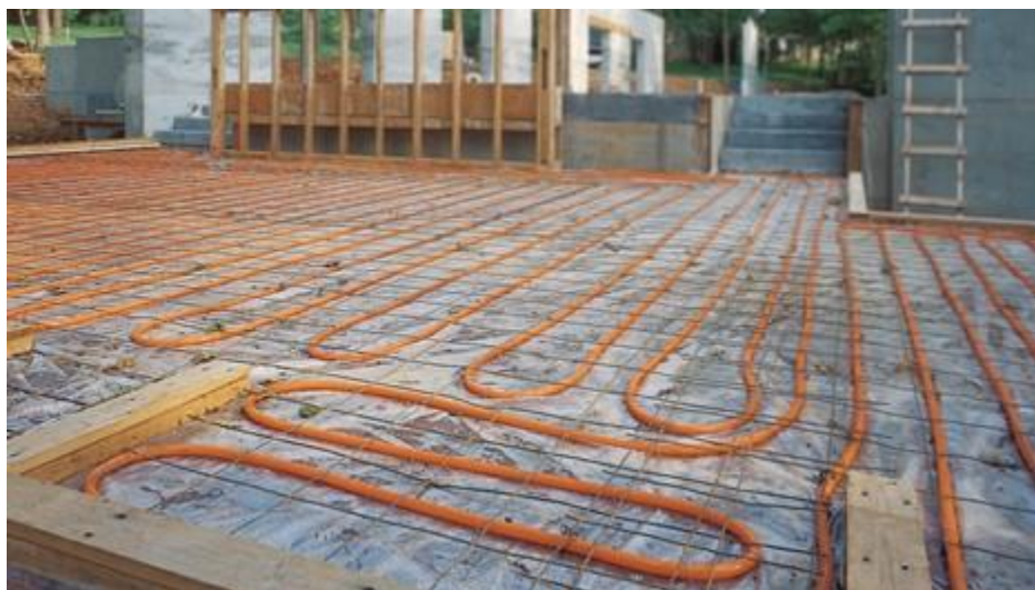
Figure 14: Underfloor radiant loop installation (Energy.gov, 2023).
