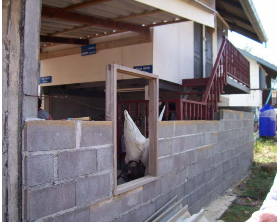
Figure 6: A cement wall addition in the middle of construction
