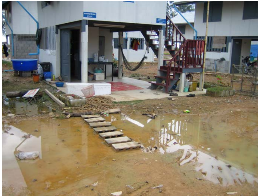
Figure 3: Water collection after light rain
