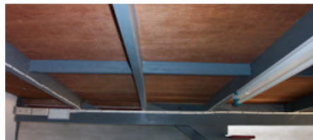
Frame of Second floor of house (painted blue)
