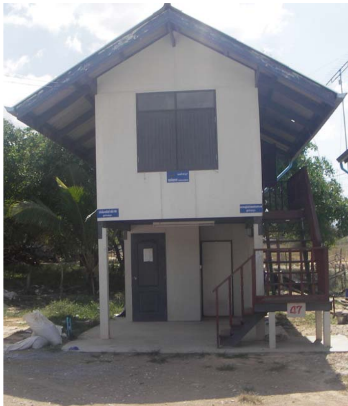
Figure 1: Replacement unit in Ranong Province, Thailand
