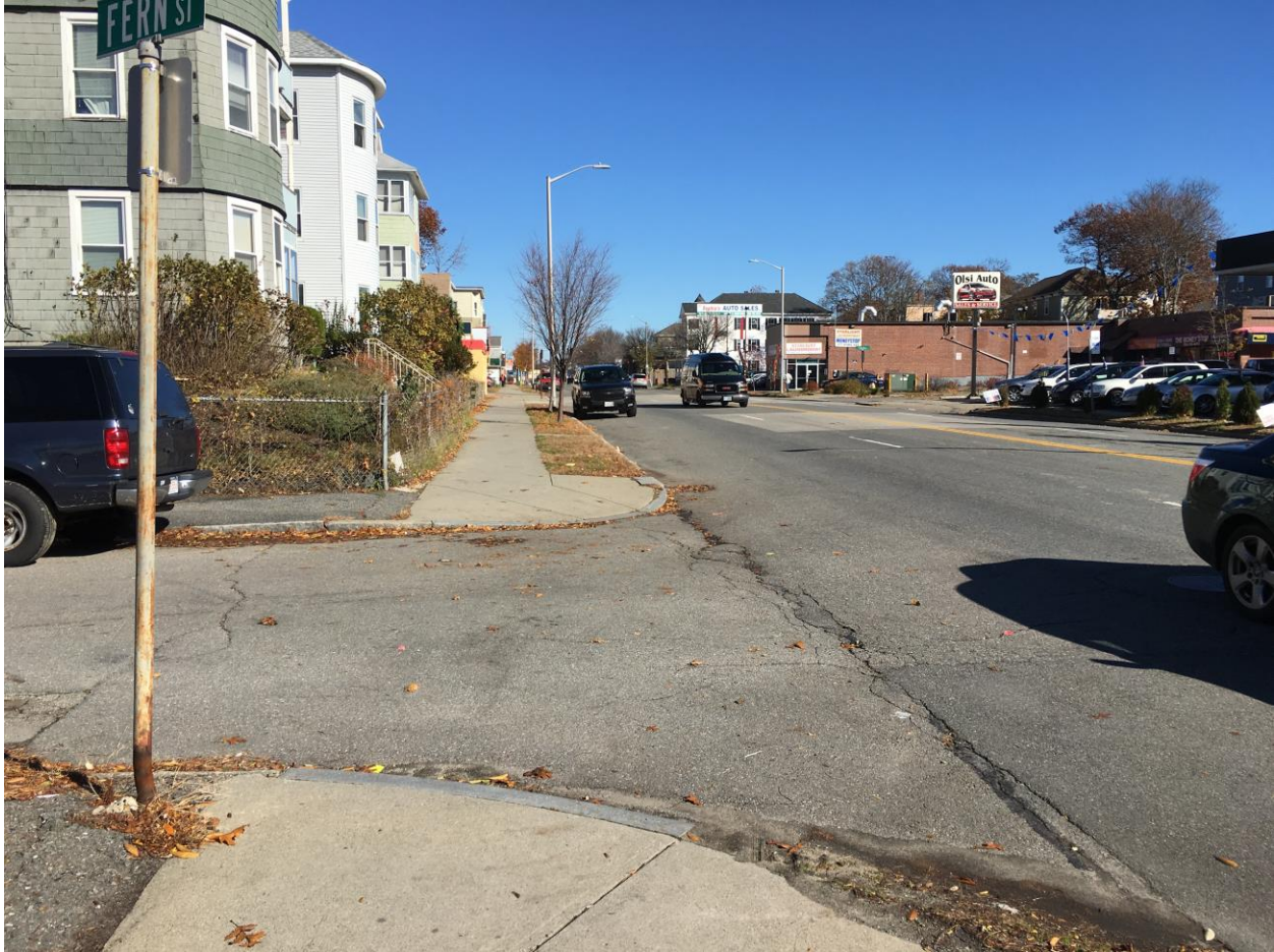
Figure 3: Photo of Park Avenue north of Maywood Street looking north (Colin Claus 11/7/18)
