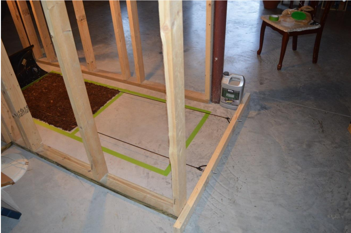
Figure 22 - Making Use of Stairwell Support for Experimental Setup
