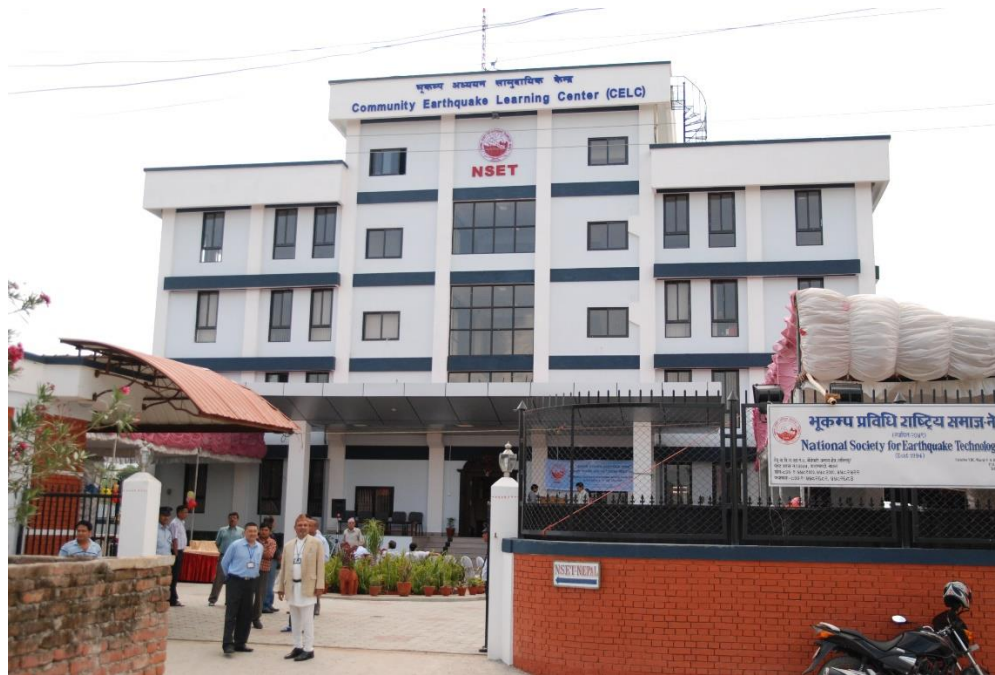
Figure 4. NSET building founded in 1993 (NSET Nepal 2009)
