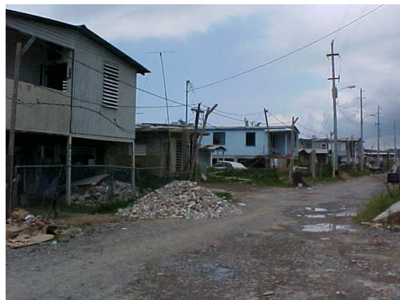
Photo 4: Unpaved Road in Villa Quintero
