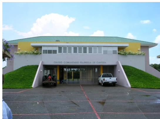
Photo 2: Cantera Community Center
