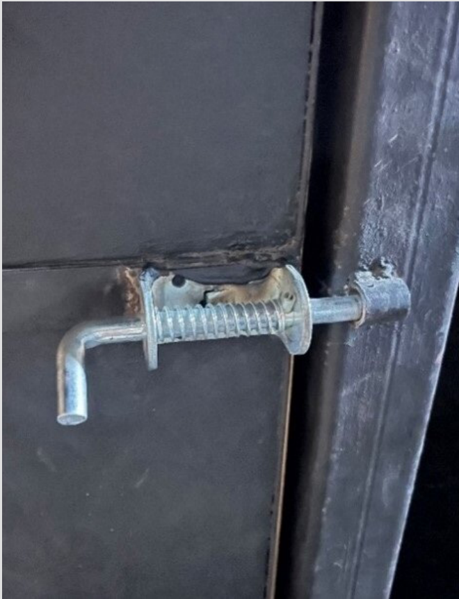
Figure 15: Picture showing a spring-loaded pin that the Bomberos currently utilize in their labyrinth design at the academy.
