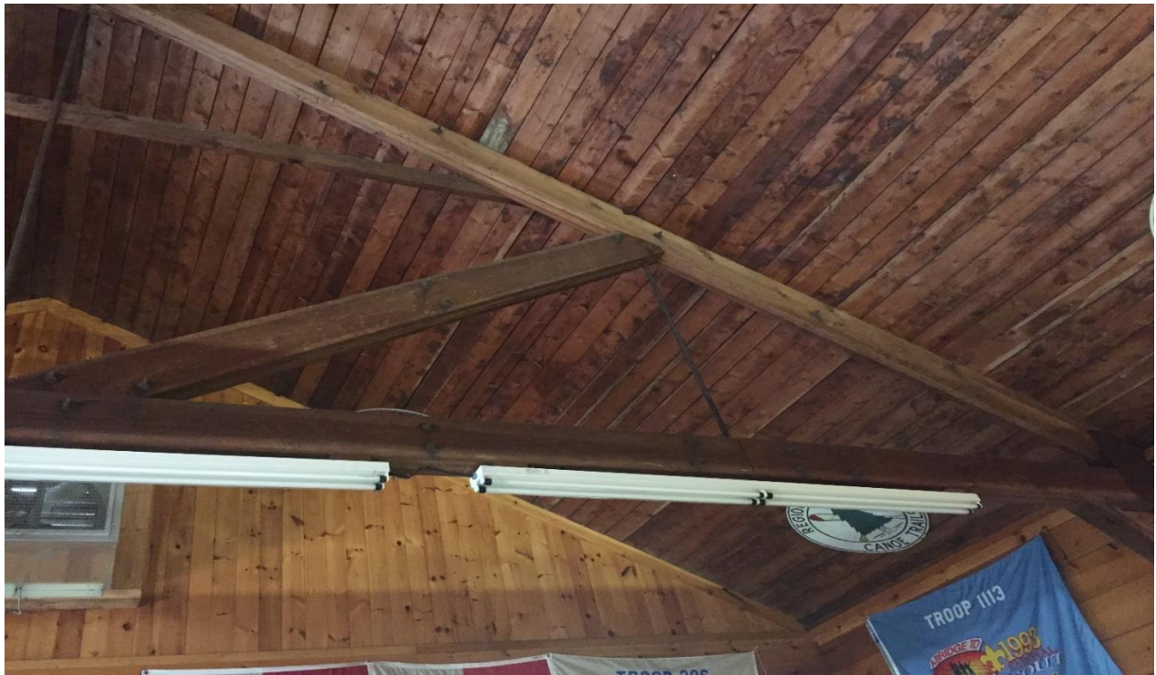
Figure: Truss structure
