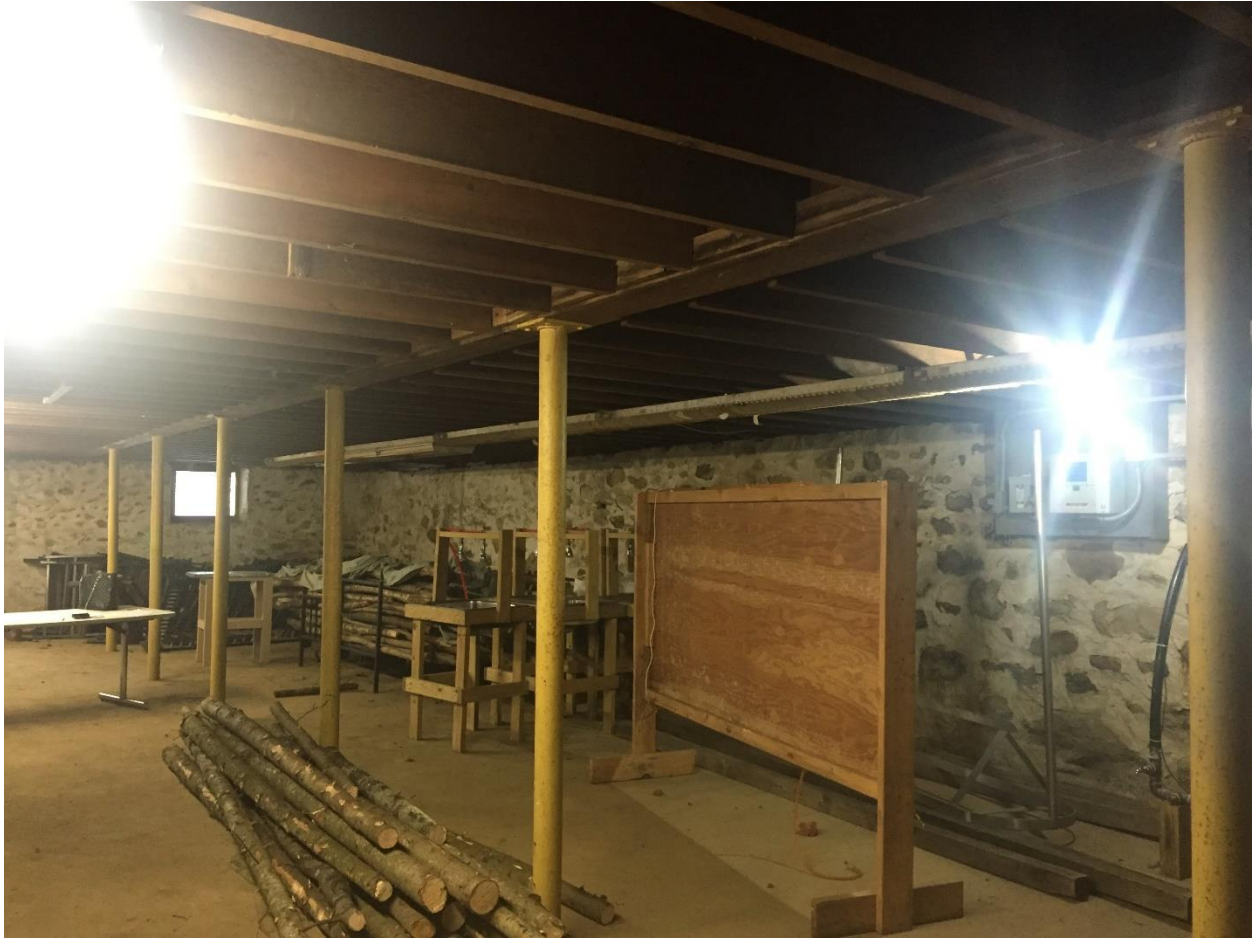
Figure 23 East Lodge basement
