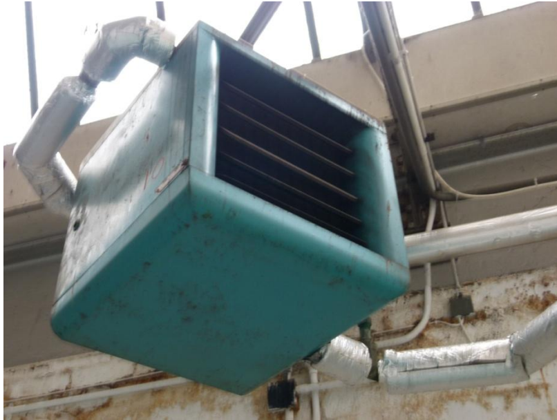
Figure 25 - Risbridger Ltd. Radiation Unit
