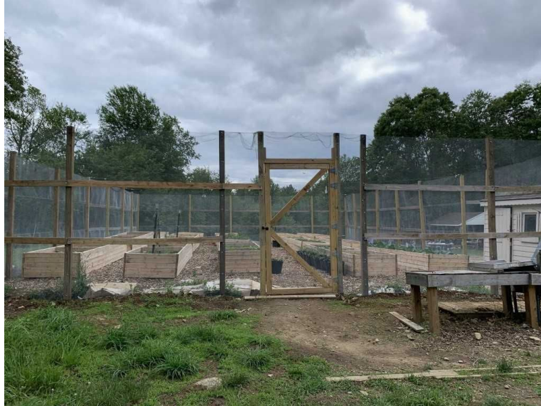
Figure 3e.iii: Final garden with 8-foot high fencing, handcrafted door, and overhead bird netting at the completion of the build process (Stoddard, 2019)
