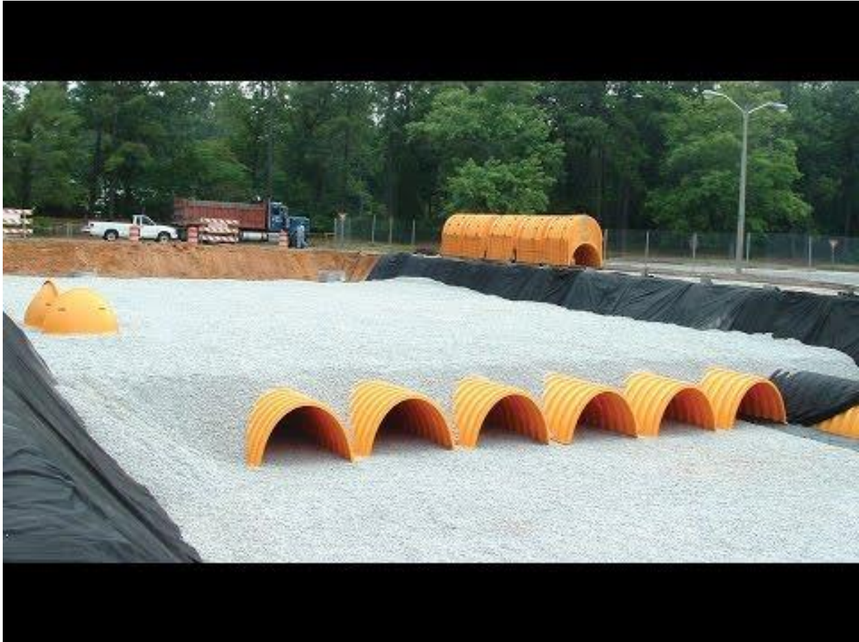
FIGURE 2: STORMTECH CHAMBERS FOR STORMWATER RUNOFF TREATMENT. PHOTO FROM ALL AROUND LANDSCAPE SUPPLY, 2016.
