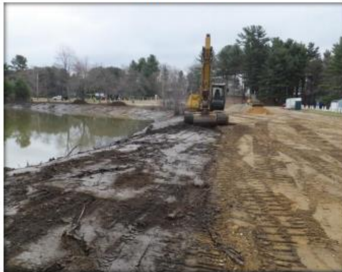
Dredging of Basin 2
