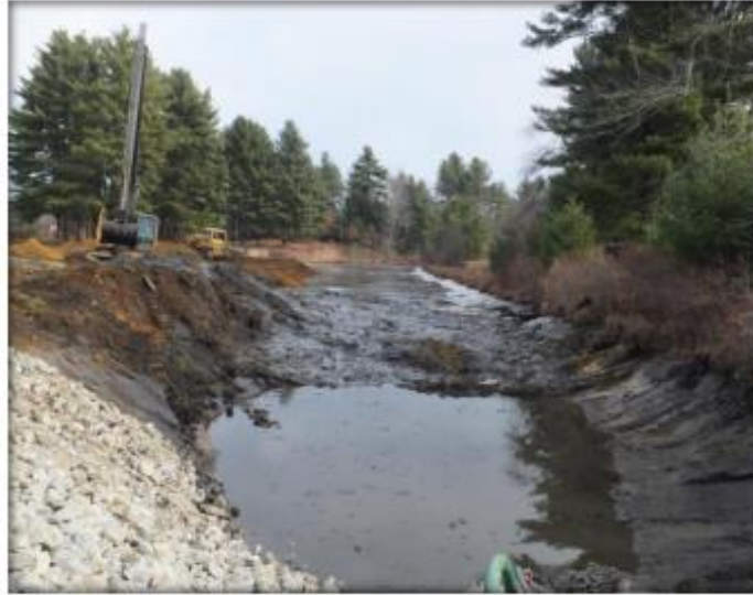
Dredging of Basin 1
