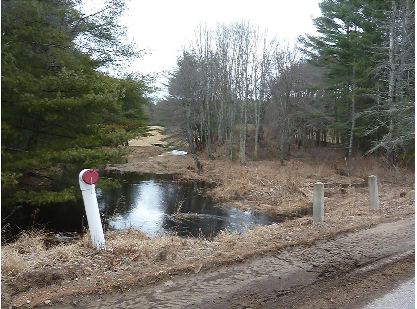
FIGURE 12: SEDIMENT ACCUMULATION ALONG SHEA ROAD AT SUCKER BROOK.
