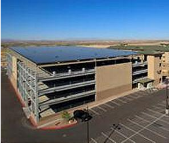
Figure 6 An Example of Rooftop Solar Panel System [16]
