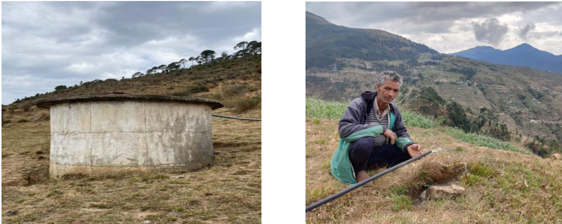
Figure 4. Water tank and open pipeline in Kundakh (Photo Credit: Manav Sharma)
