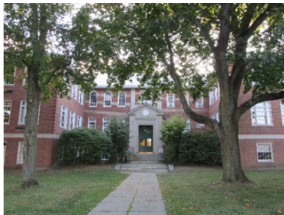
Figure 1 Existing Kaven Hall
