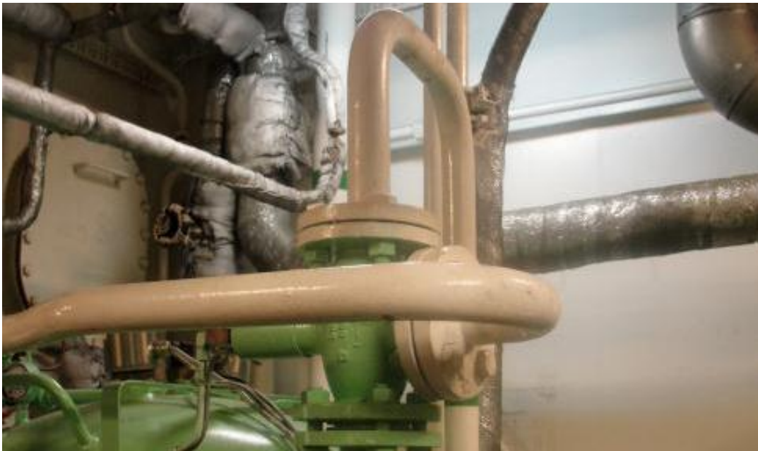
Figure 11: Outflow Valve
