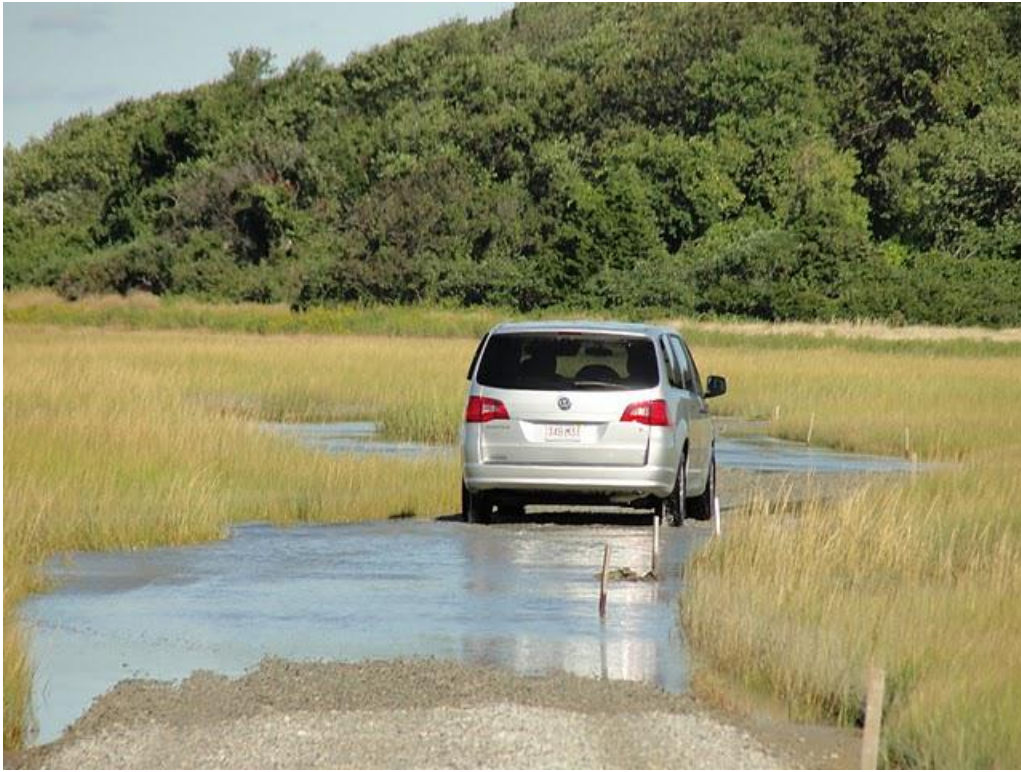
Figure 43. Flooding of Macomber's Way on September 16, 2011 (Photo source: Brendan Stitt)
