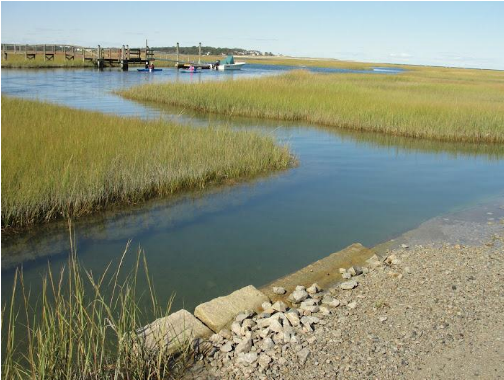
Figure 39: Uneven flooding conditions near Stone Blocks (Stitt, 2011)
