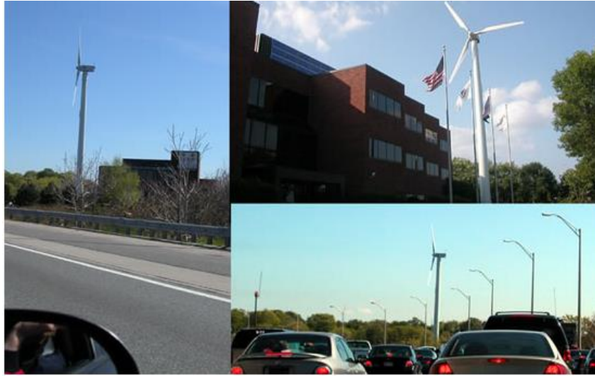
Figure 4. Wind turbines in Boston, MA
