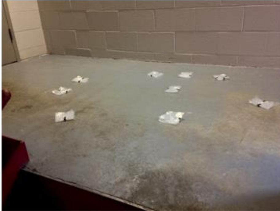
Figure 4. One of the landings in the stairwell covered with land mines.
