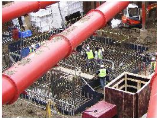
Rebars and caps on site
