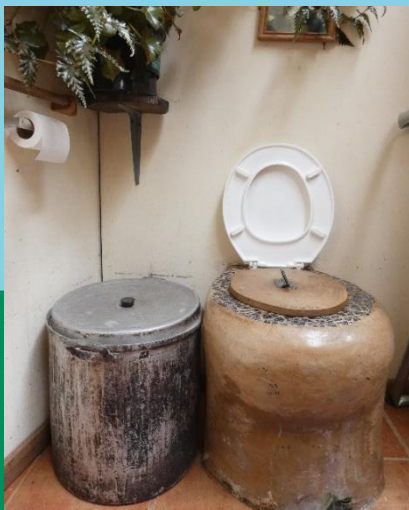
Examples of composting toilets already installed in Monteverde.
