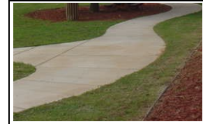
Figure 24: Sidewalk – Above Average Condition
