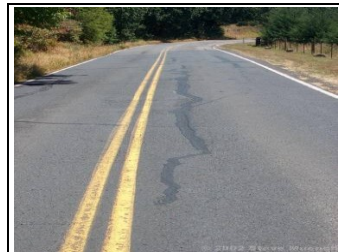
Figure 10: Paved Road - Average Condition
