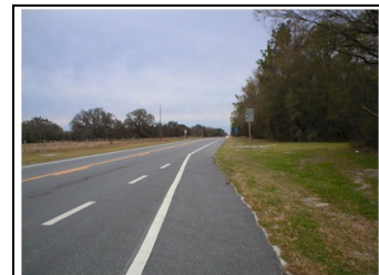
Figure 8: Paved Road - Excellent Condition
