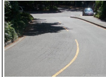
Figure 9: Paved Road - Above Average Condition
