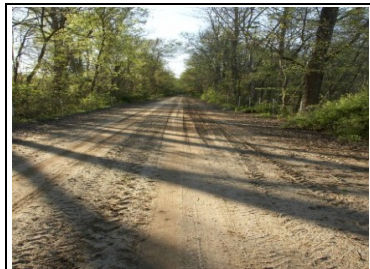
Figure 16: Unpaved Road – Below Average Condition
