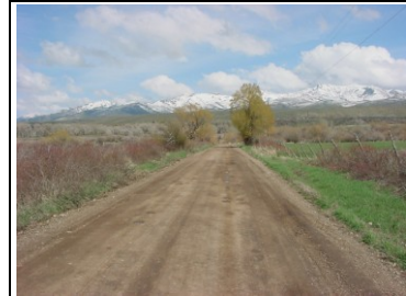
Figure 15: Unpaved Road – Average Condition
