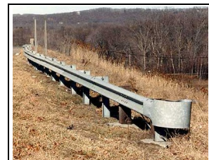
Figure 29: Guardrail – Average Condition
