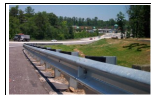
Figure 28: Guardrail – Excellent Condition
