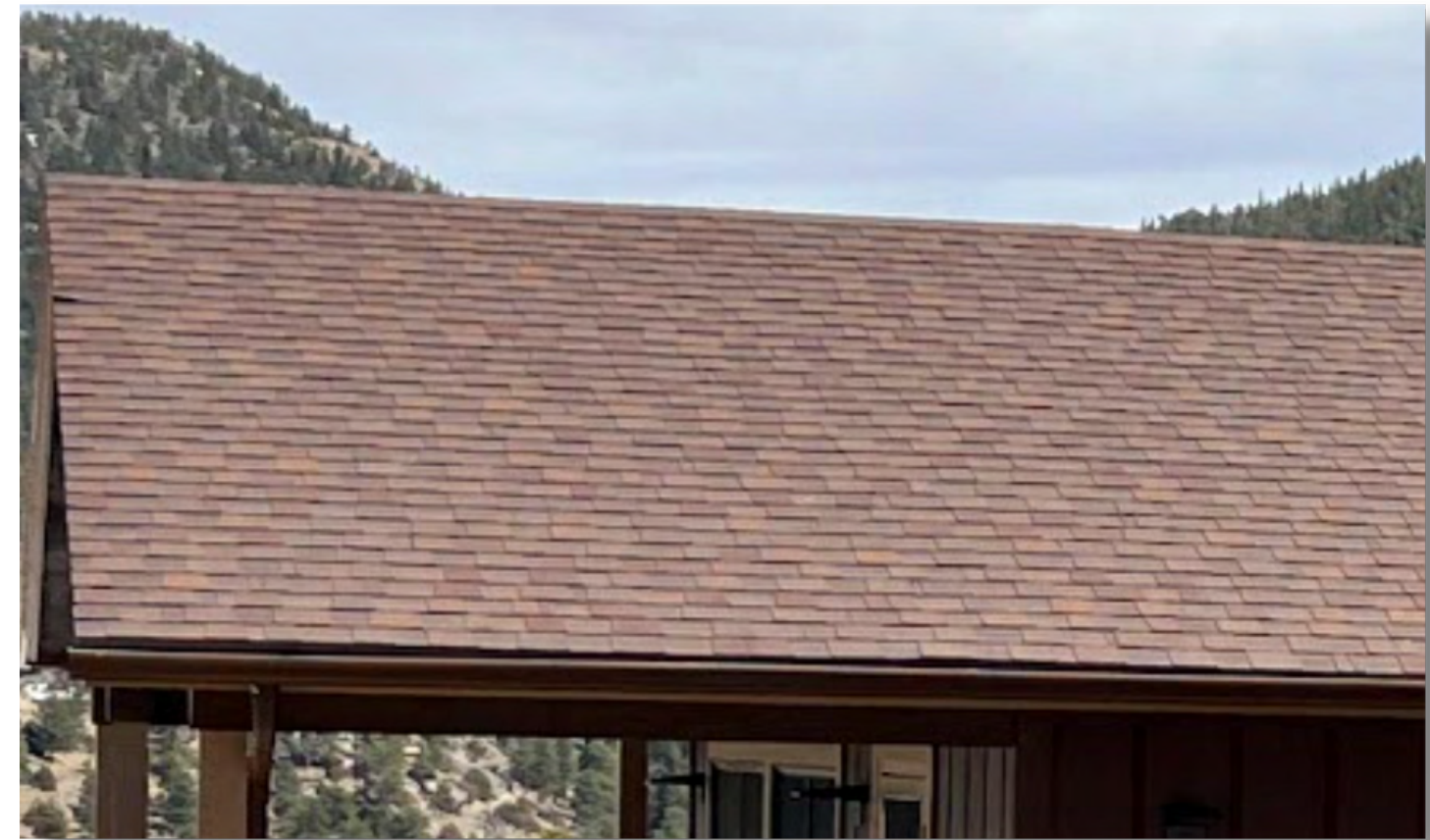
Figure 21: Image of Architectural Asphalt Shingles at the YMCA.
