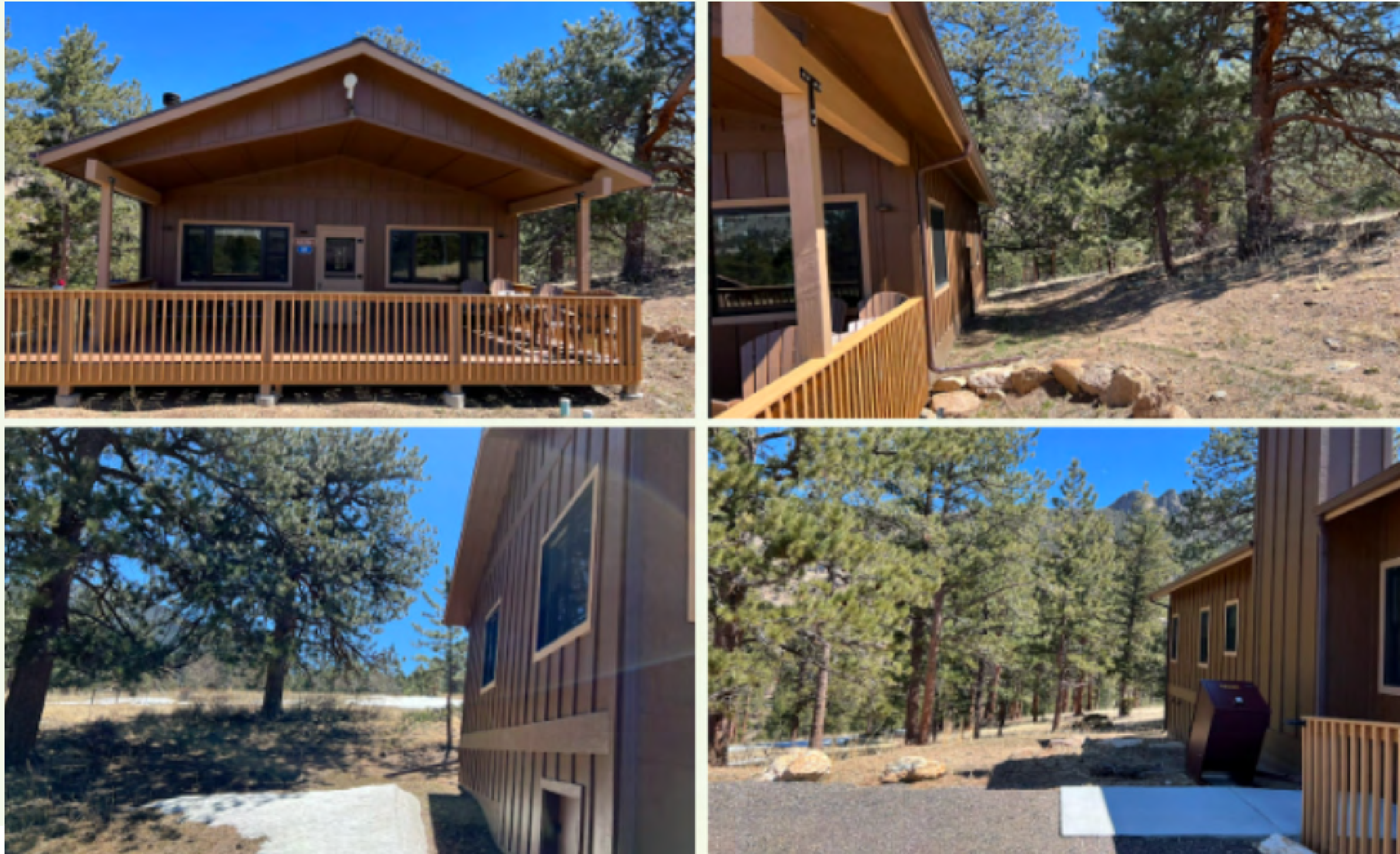
Figure 28: Images of Black Bear, a low risk cabin. Note how there is no vegetation surrounding the cabin within 5 feet, no gutter debris, and no overhang.
