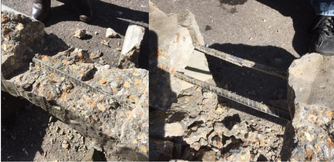
Figure 15. Concrete stop broken to expose rebar.
