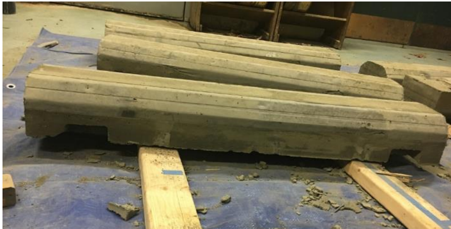
Figure 11. Concrete stop after 24 hours with breaks in hand holds.
