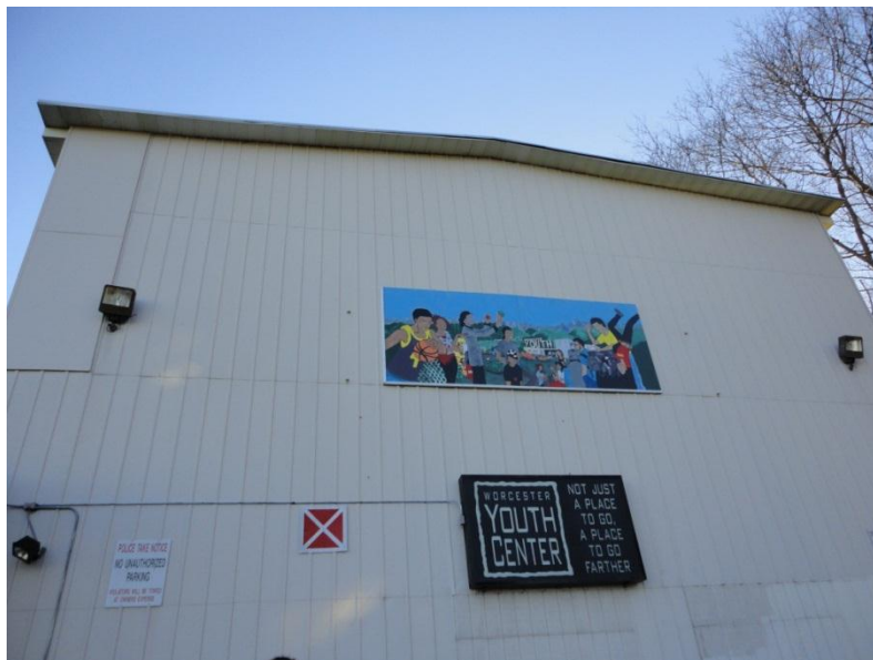
Figure 6: Front view of the warehouse
