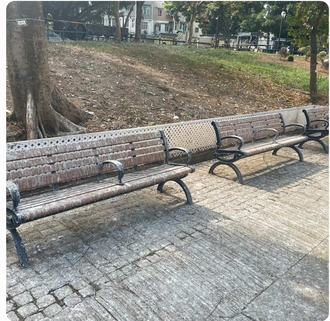
Figure 21: Benches on Lam Tsuen River Waterfront covered in bird droppings.
