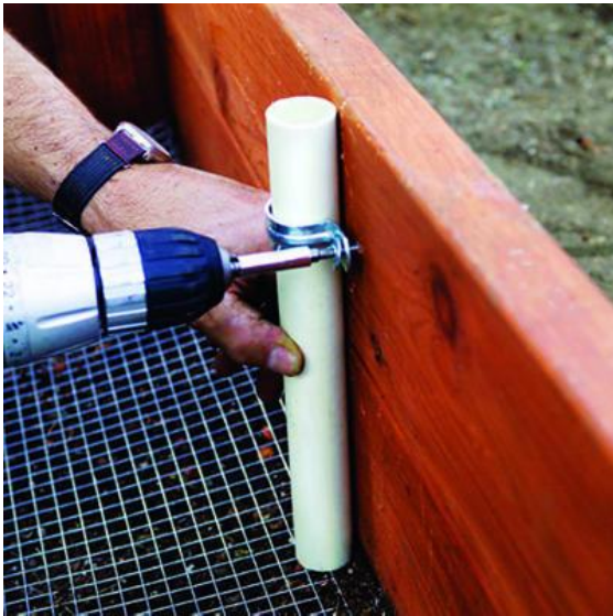
Figure 3.4: Mounting a frame holder.
