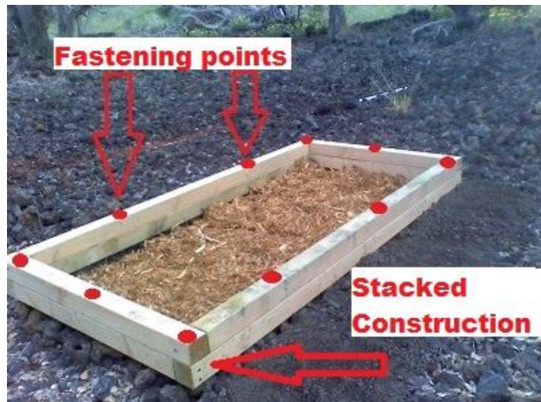
Figure 3.3: Fastening points (all rows after first)
