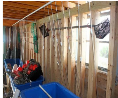
Figure 74: Rebuilt wall frame in Shellfish Lab
