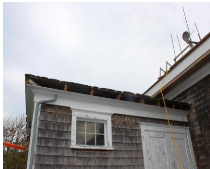
Figure 72: Roof construction at Siasconset Fire Station
