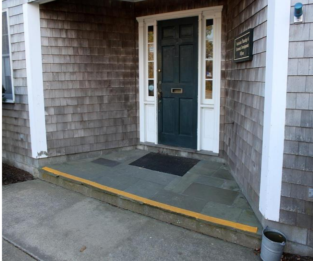
Figure 19: Large step at entrance of PLUS
