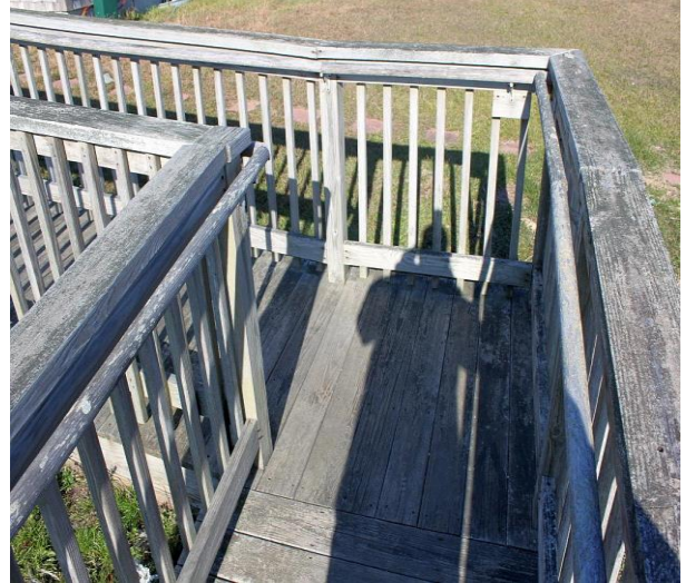
Figure 20: Tight ramp at DPW Administrative Building
