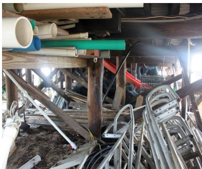
Figure 78: Cluttered storage space
