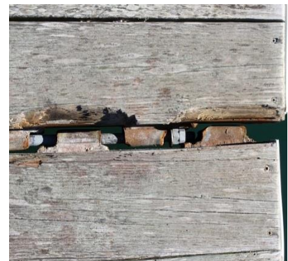
Figure 46: Rusting connections
