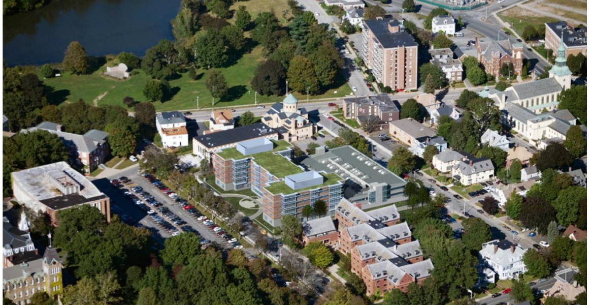
Figure 6-1 Aerial view of WPI Residence Hall on Boynton Street
