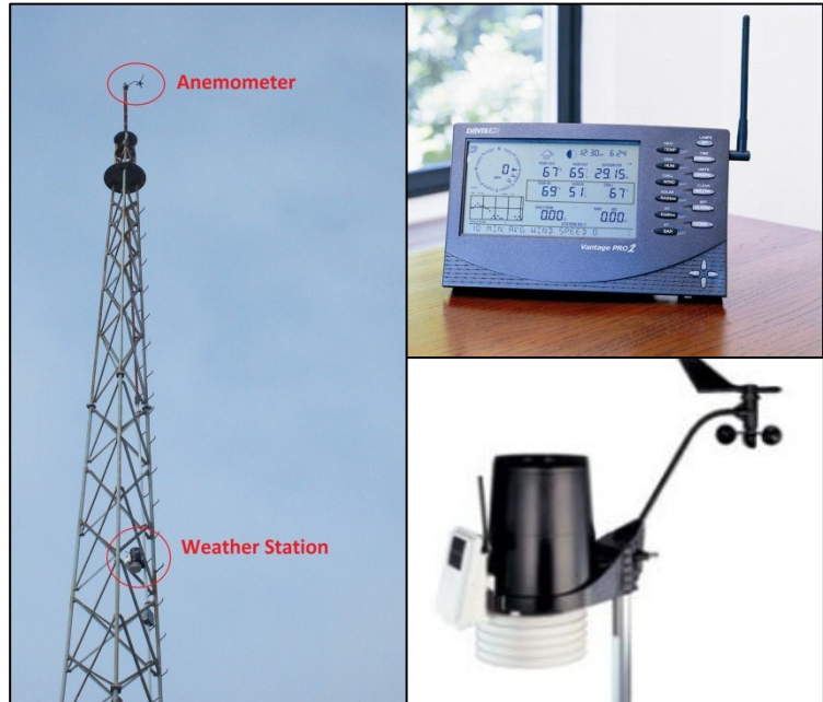
Figure 8: The Davis Instruments Vantage Pro II (top & bottom right) and the EcoTarium’s radio tower after installation (left) (Image credit: Davis Instruments)
