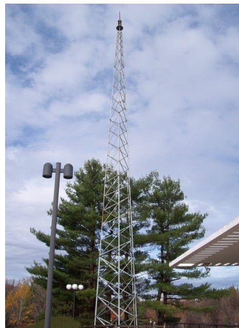
Figure 2: The EcoTarium's radio tower, complete with anemometer and weather
