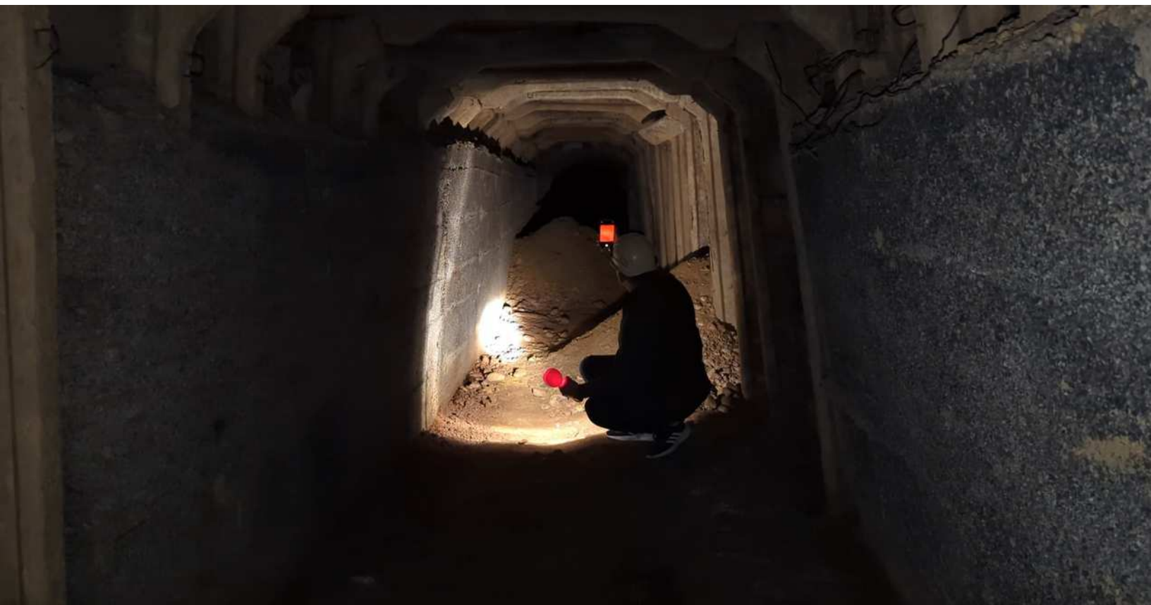
Image 5: Andrit Shehu scans a collapsed section of the underground city
