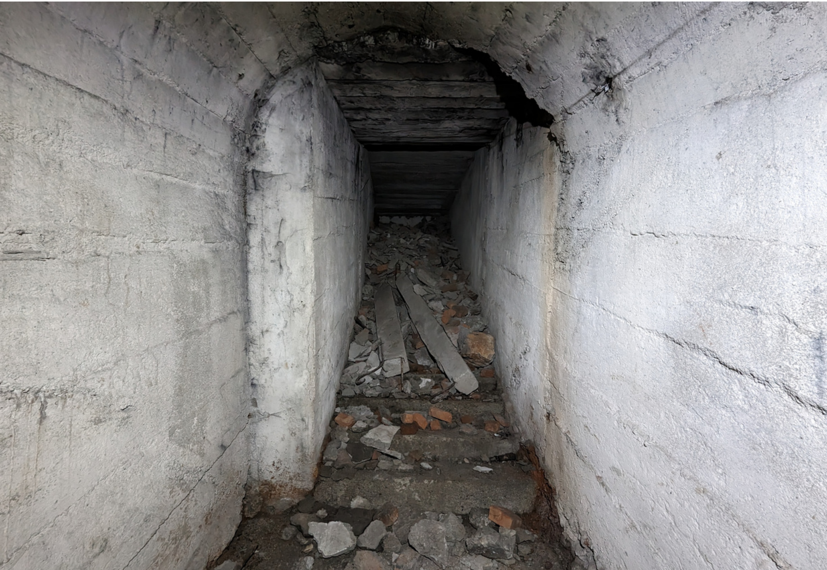
Image 23: Barricaded entrance to tunnels
