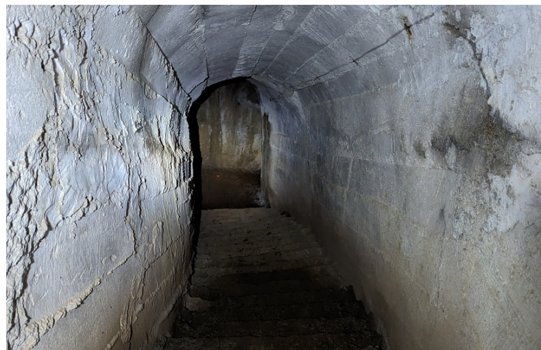
Image 4: Underground tunnel in Kukës
