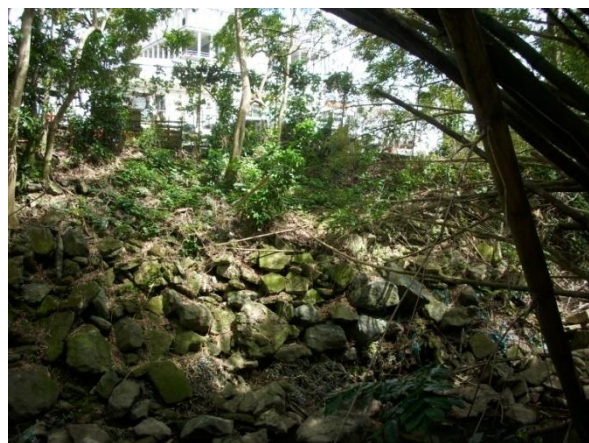
Figure 17: Rock Embankment of Zone 5
