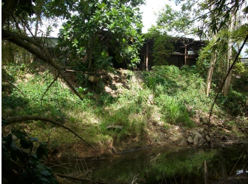
Figure 15: Zone 4 River Bank and Building
