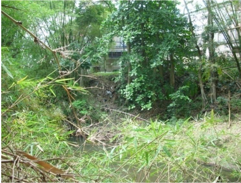
Figure 14: View of Zone 4 from Aqueduct Side, Building and Fence Present
