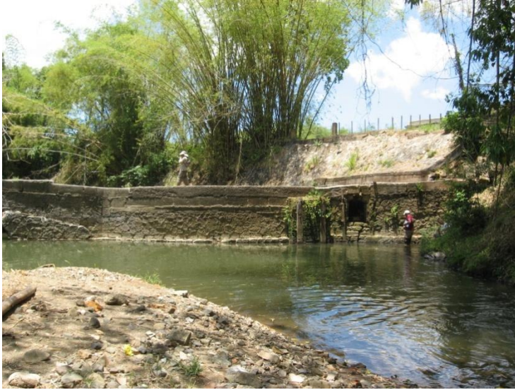
Figure 23: End of Zone 7 at the Aqueduct
