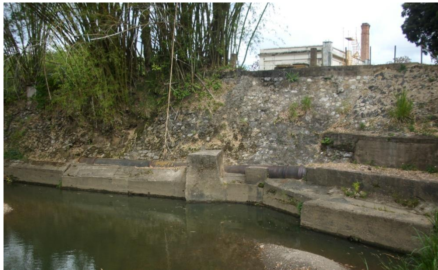
Figure 24: Aqueduct Concrete Wall of Zone 8
