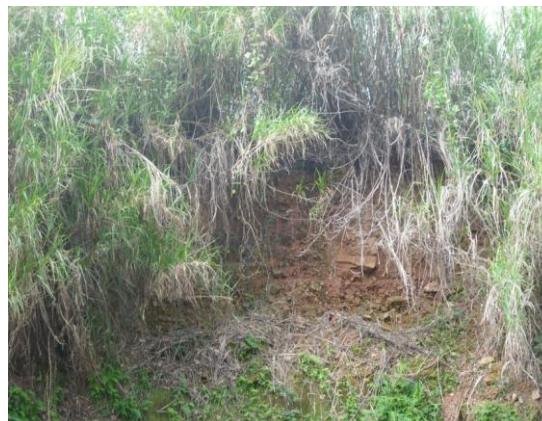
Figure 21: Erosion in Zone 1
